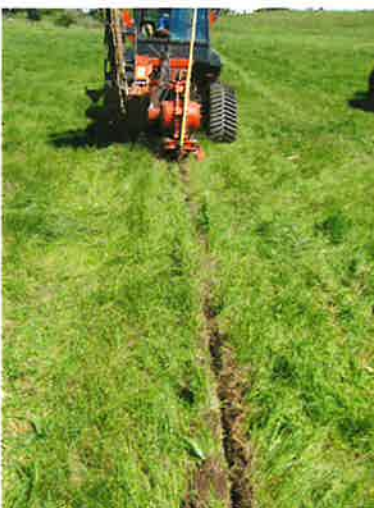
Typical installation of a pipeline.
