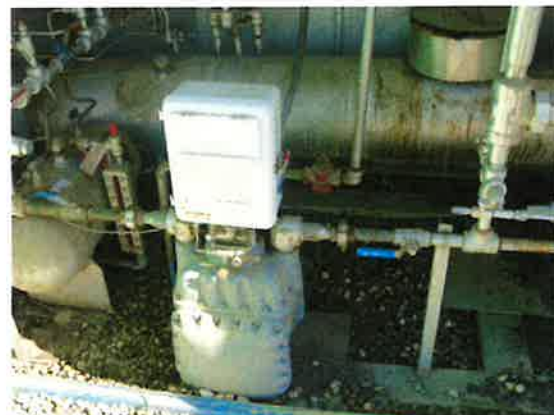
Interior of second type of RMO station.
