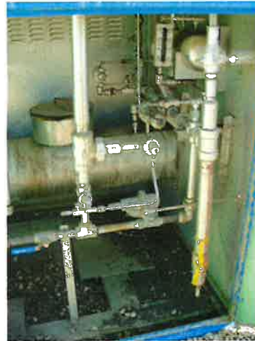
Interior of second type of RMO station.
