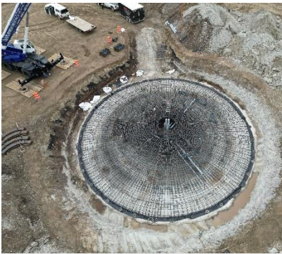
An aerial view of the reinforcing steel rebar.
