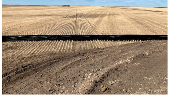
Erosion control measures along edge of a turbine pad under construction
