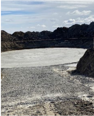
A concrete seal slab is poured in the excavated foundation prior to the reinforced rebar being installed for the concrete foundations.
